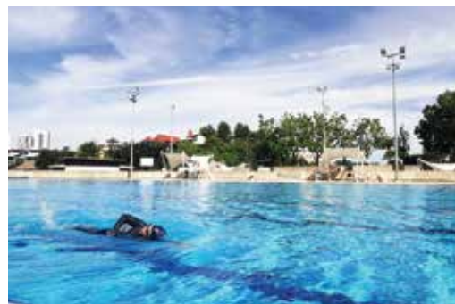
Swimming Pool at Neighbourhood Community Centre
